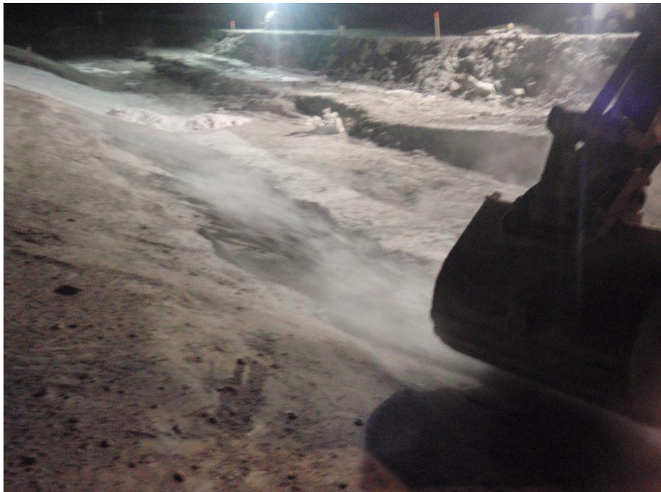
Photo 10: View of 330 bucket spreading FCM in underbuilt upstream slope area around station 1+20.
