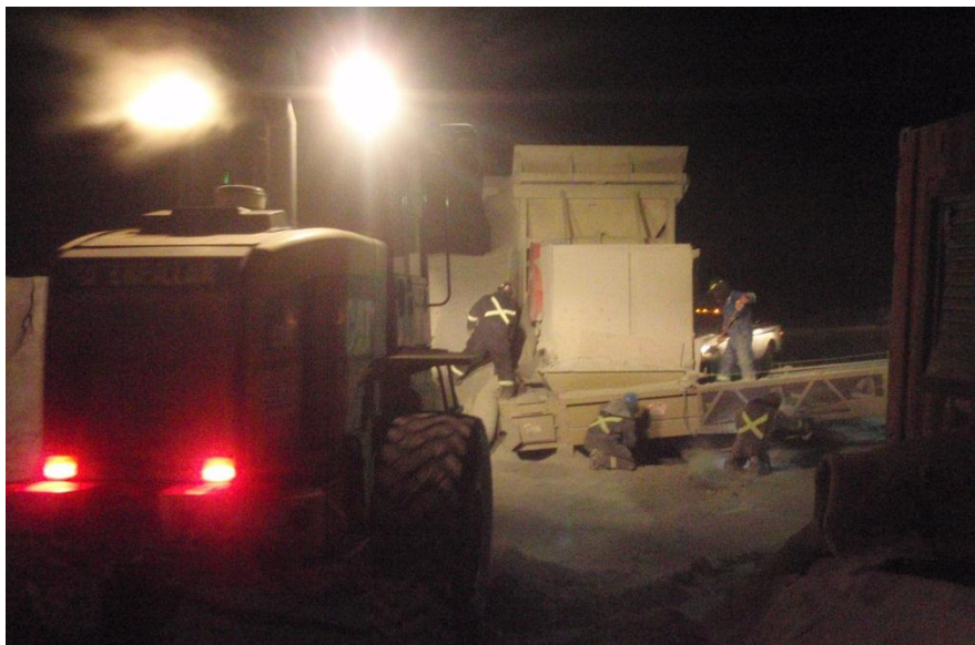
Photo 14: Labourers, supported by the loader, digging out feeder and Grizzly at the Frozen Core plant.
