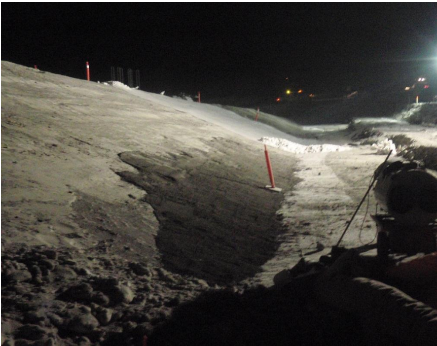
Photo 11: View of completed placement around 1+20. This placement was completed to fill in the previously underbuilt toe. area.
