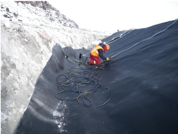
Photo 7: Welding of liner on diversion berm, photo looking east.
