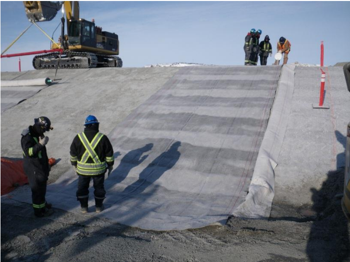
Photo 6: Placing bentonite on GCL seam. Note the striped colouration of the GCL.
