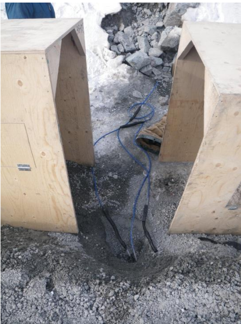
Photo 4: Thermistor cables at 1+75 after splicing.
