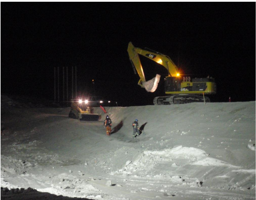
Photo 9: ~ NNW view of SSE underbuilt upstream slope area after cleaning activities had resulted.
