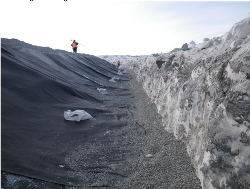
Photo 5: Looking west along diversion berm key trench. Bentonite 'plug' on right side of photo.
