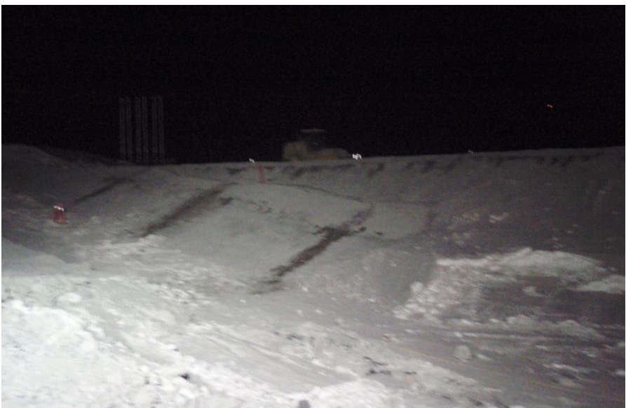
Photo 13: ~ NNW view of SSE underbuilt upstream slope area, after today's placement. Note some water that bled / ran down the side slopes in areas.
