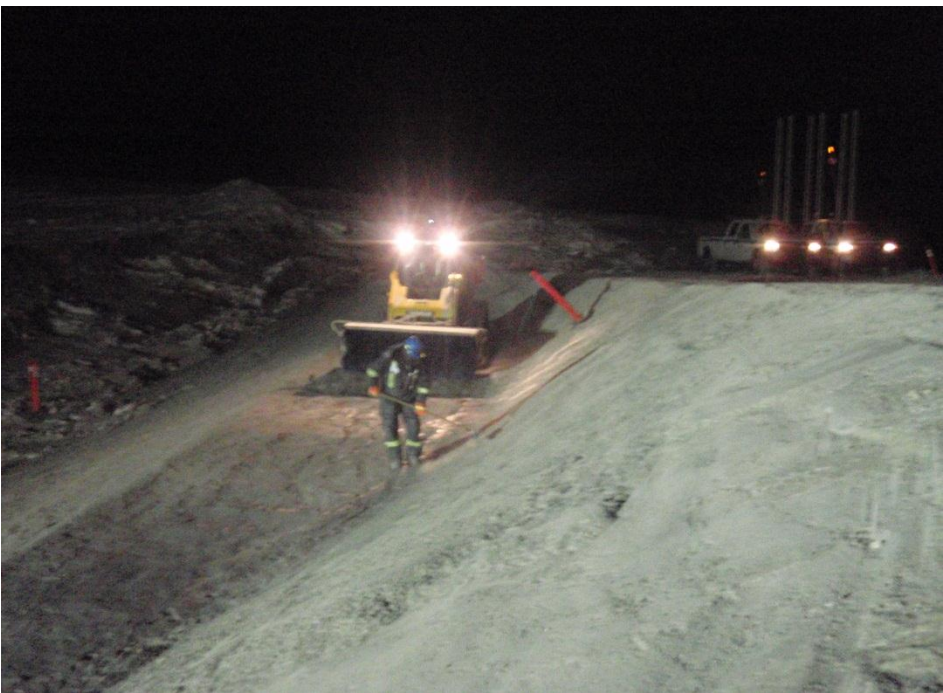
Photo 8: ~WSW view of cleaning activities in the SSE underbuilt core slope area (Station 0+40 to 0+70)
